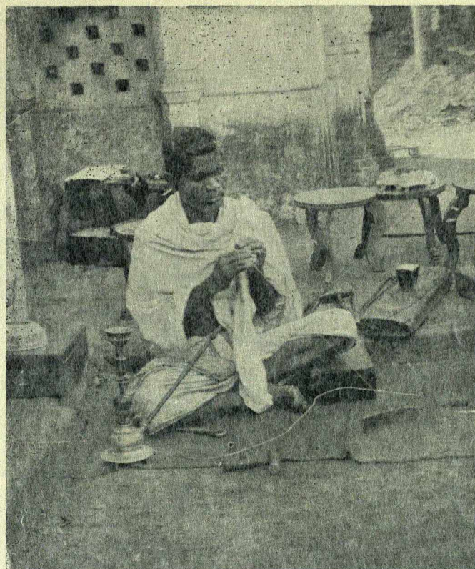
Wire Twisting for Filigree Work—CUTTACK.
