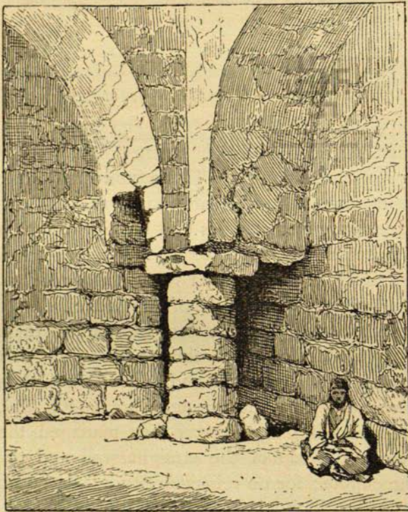
FIG. 85.—Sarvistan. Column and springing of the arches of one of the halls. Ibid. , Plate VI.
