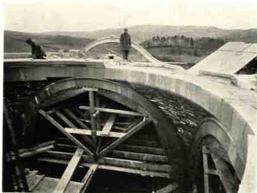
THE DOME IN CONSTRUCTION
