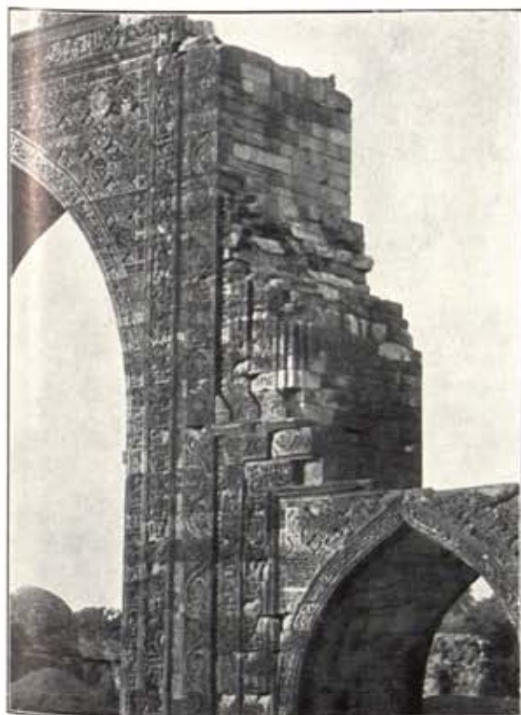
(c) QUTBU-D-DIN'S ORIGINAL SCREEN. DETAIL VIEW OF BROKEN JAMB OF UPPER SUBSIDIARY ARCHED OPENINGS (NOW MISSING). SEE DRAWING IN PLATE No. IV FOR RESTORATION OF SCREEN.
