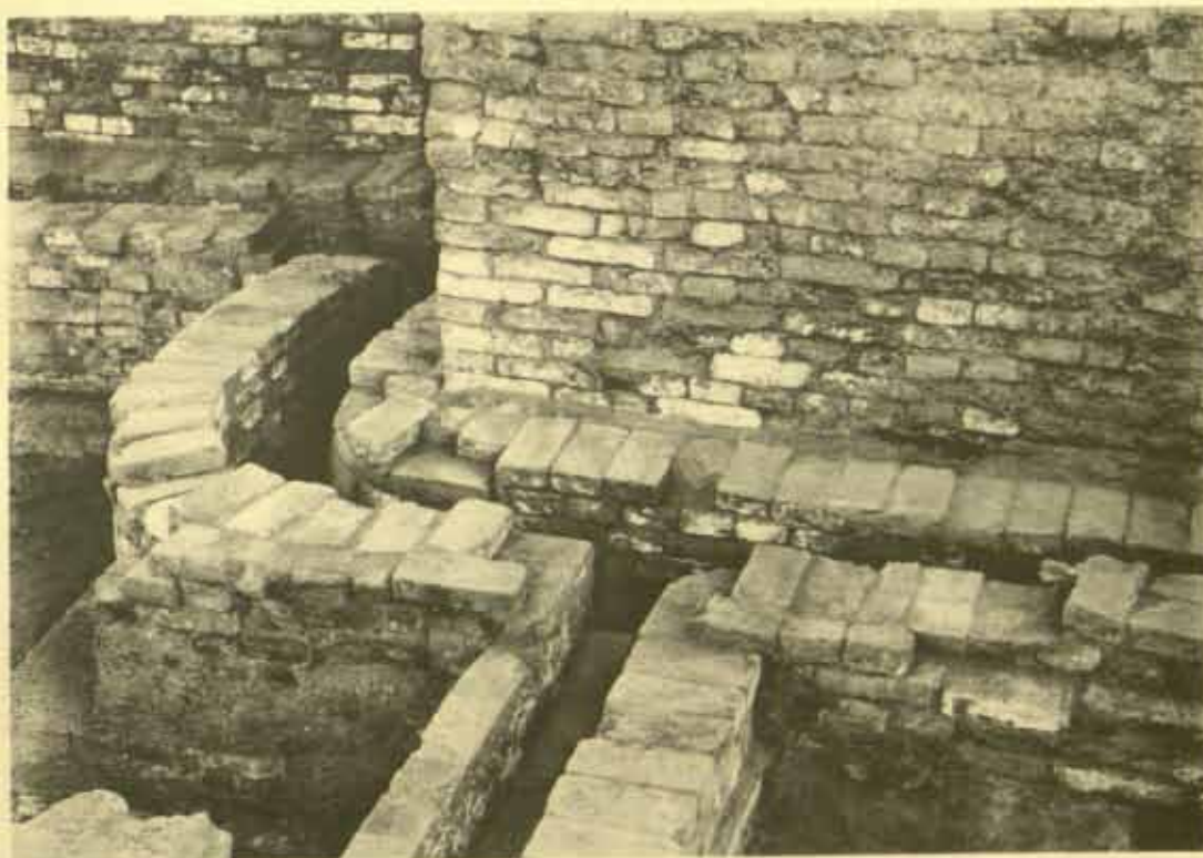
a) SD. Area. Drain with curved corner.
