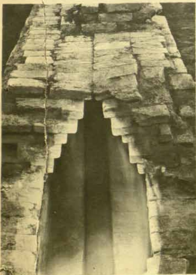
c) Culvert in HR. Area.
