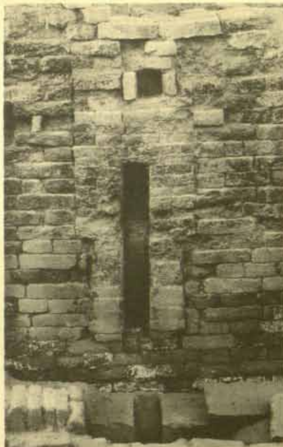
b) Water-chute in street, Section C, DK. Area.
