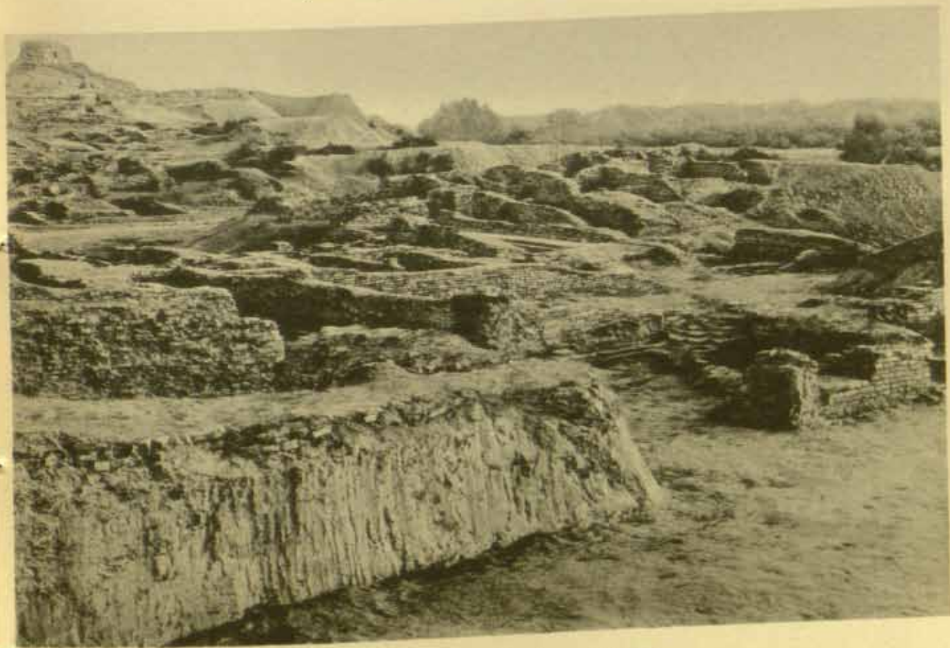
b) Section C. Block 4 and 5, from south-west.
