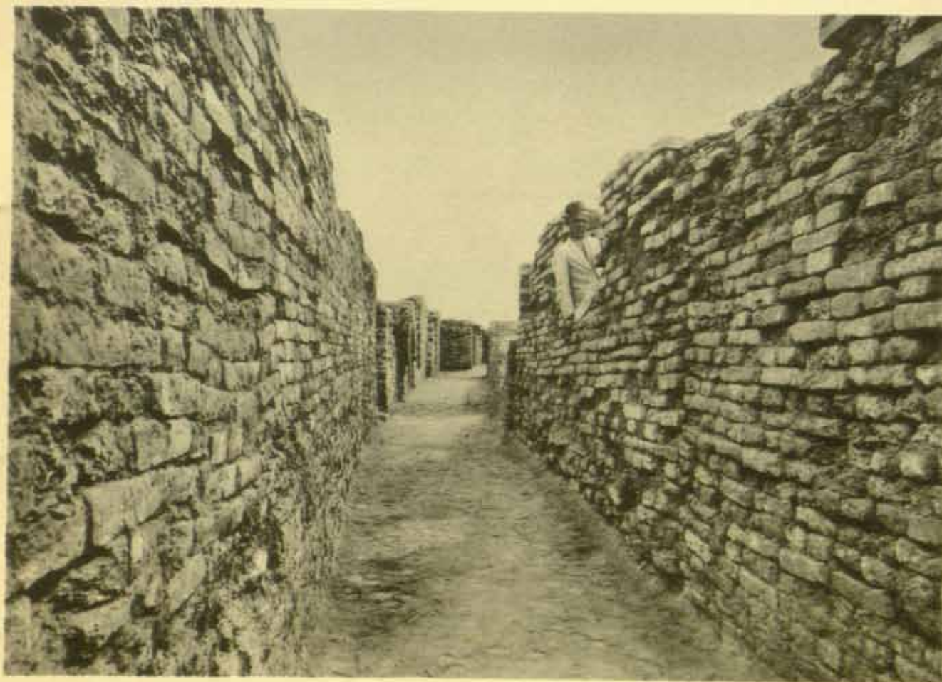
b) South Lane, looking east.
