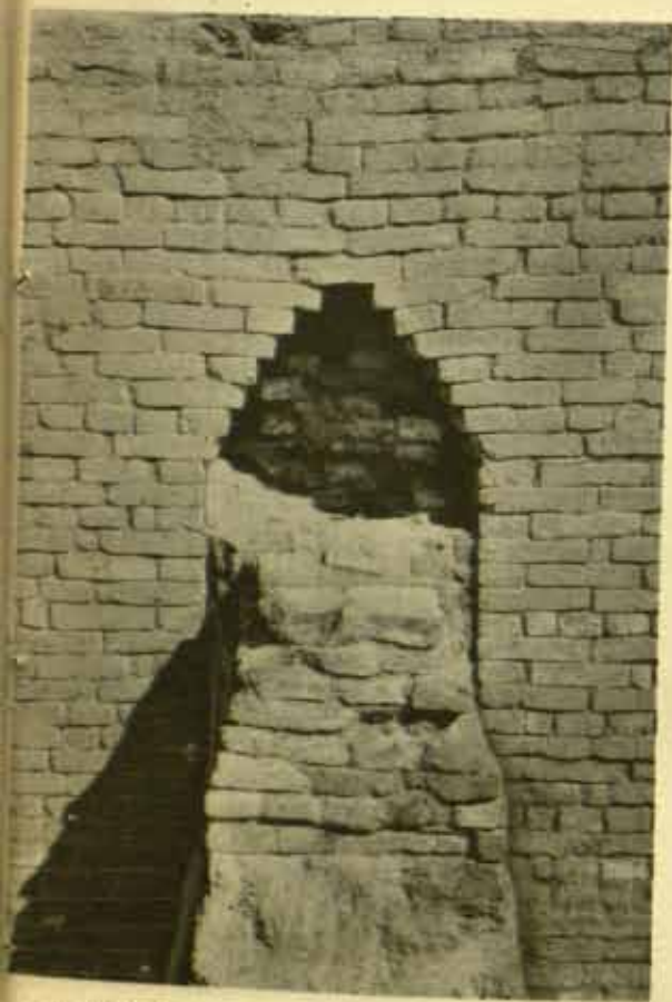
b) HR. Area, Section B. Block 2, House V: Corbelled arch between Rooms 49 and 54.
