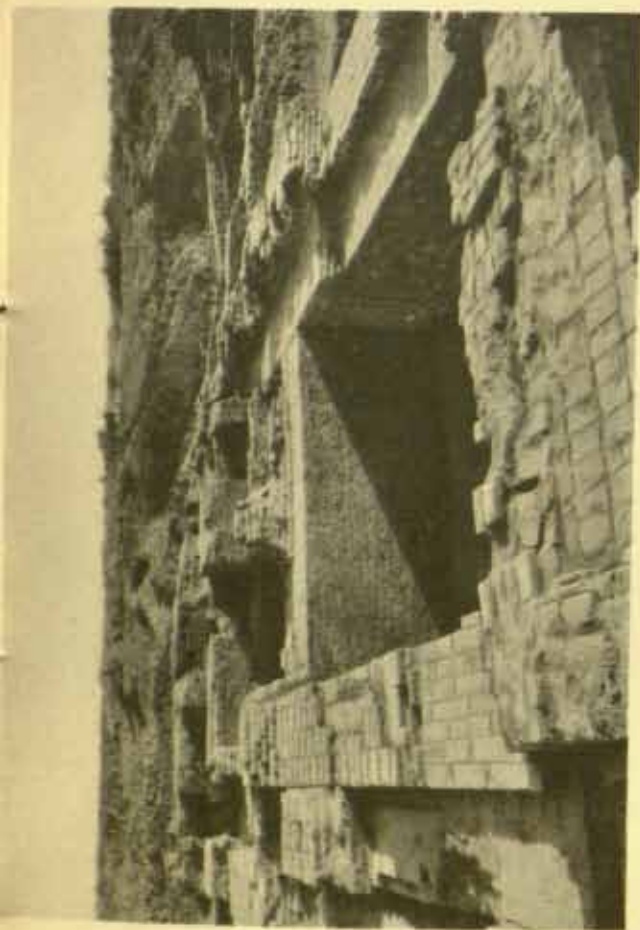
a) Block 5, Building XXX, showing deep foundations.
