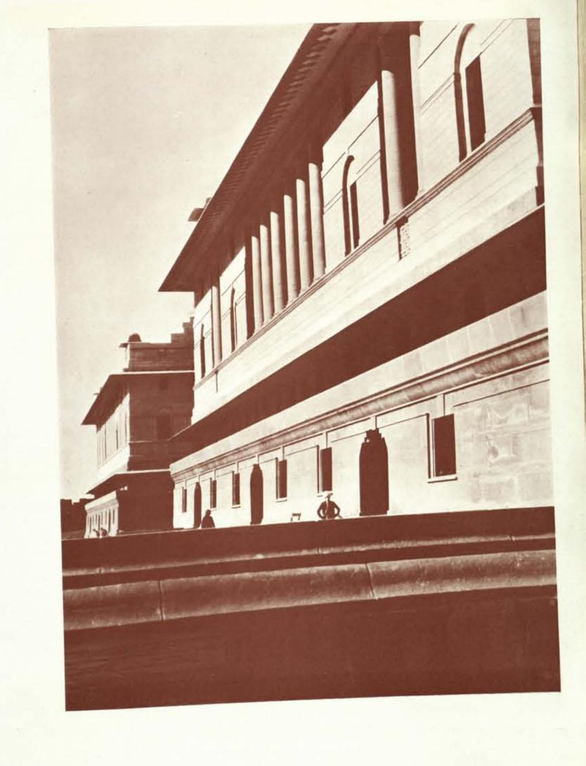
A detail of the south front of the Viceroy's House, showing the pattern beneath the chujja (cornice), the lower chujja and gallery, and the extra foundation necessitated by the ground level.
