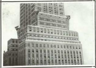
Here is an example from the U.S.A. The Chrysler building in New York is an illustration of the use of Cast Aluminium for external decoration. The Spandrels or Wall Panels, and numerous other fittings of ornamentation and practical utility, are of Cast Aluminium. For this class of work Cast Aluminium shows many advantages. It is most attractive in appearance, needs no painting, forms no stain on adjacent materials, is light and easy to erect.
