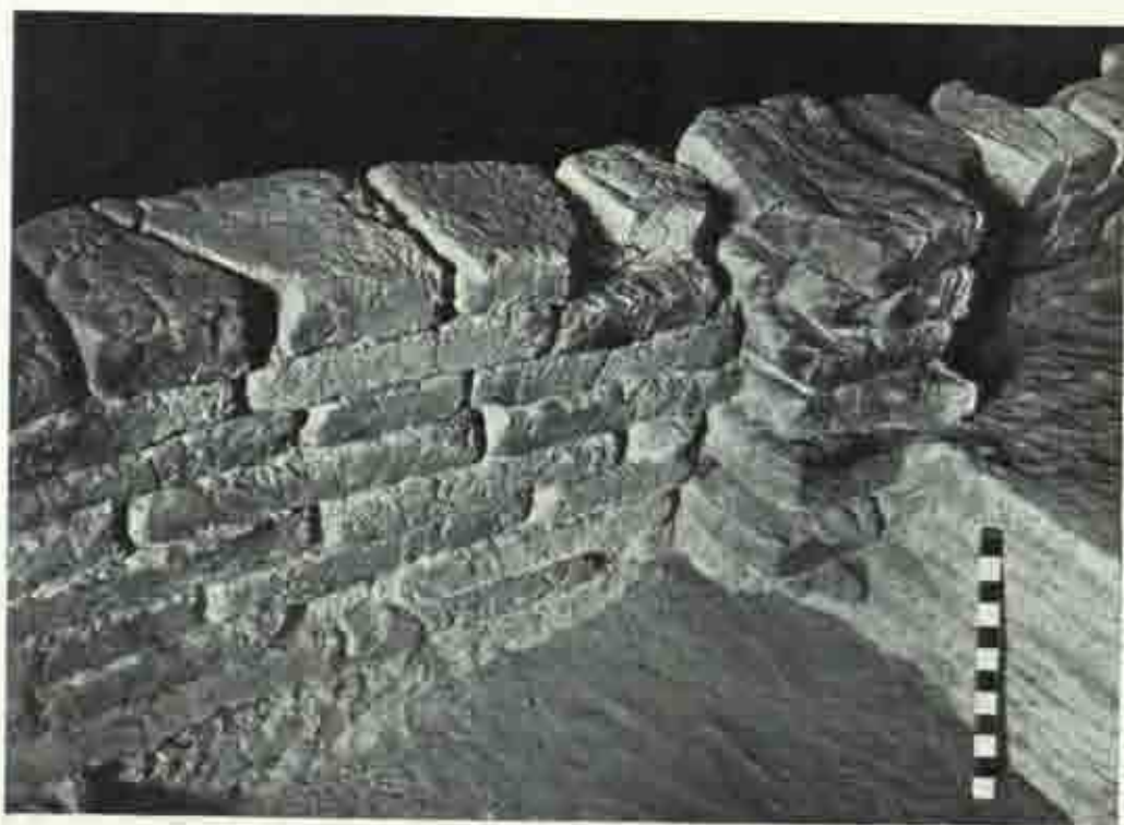
B. HST 1: retaining wall 63, showing projection for bonding, Period III (see page 25)
