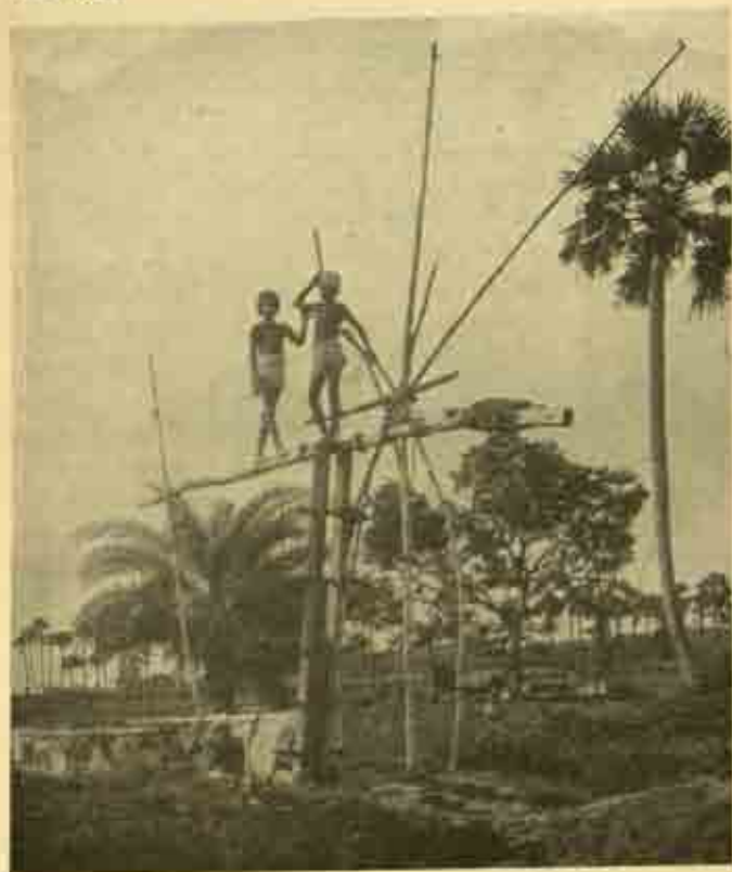
Fig. 70. Lifting water by means of a picota.
