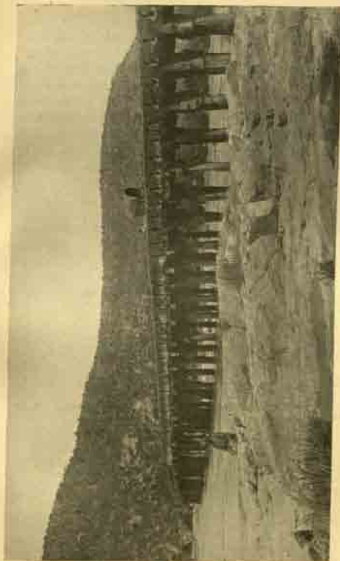
Fig. 27. Bridge made of slabs of gneiss split by fire.
