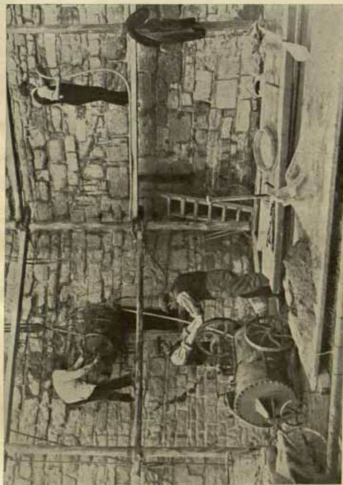
GROUTING MACHINE AT WORK (SEE PARA. 147).
