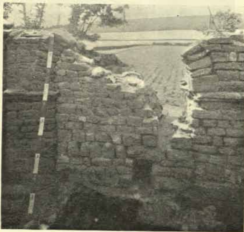
Fig. 4. Internal view of the South Gate.
