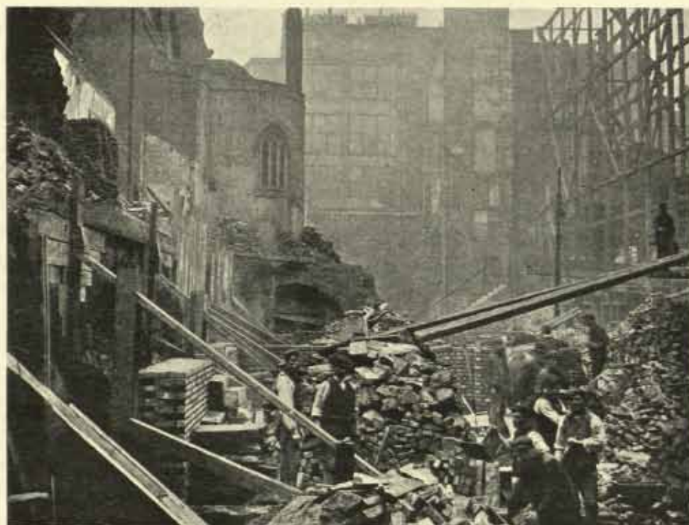
Fig. 14. Photograph showing site of City Ditch excavated.
