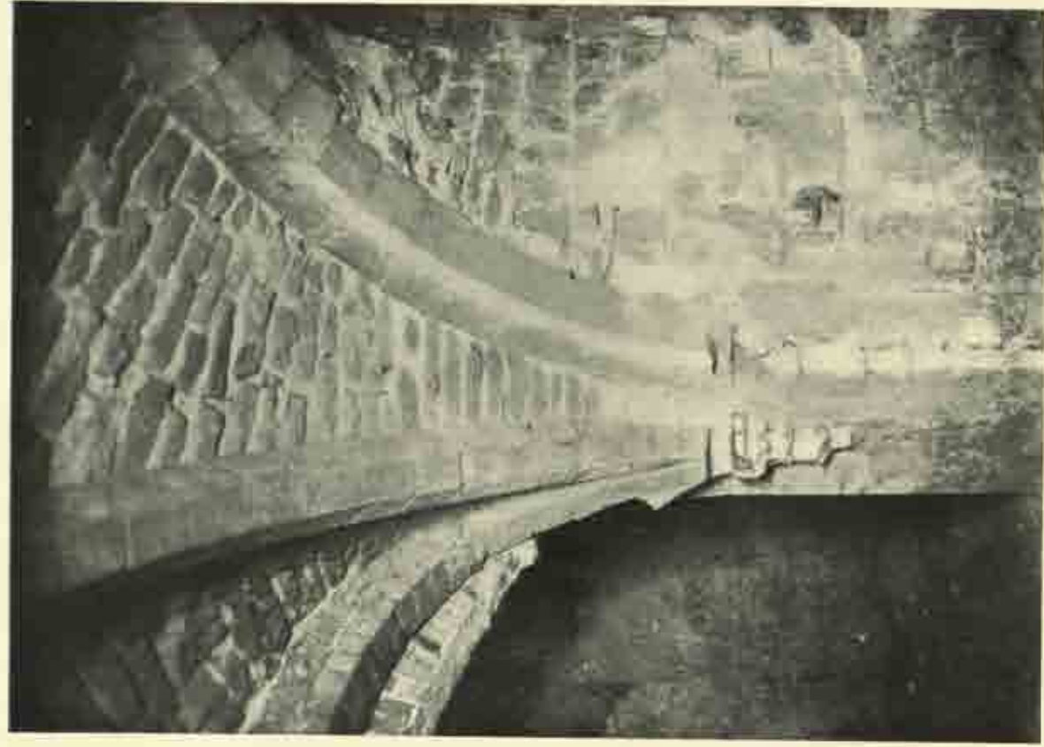
Fig. 2. Springing of vaulting, reredorter subvault.
