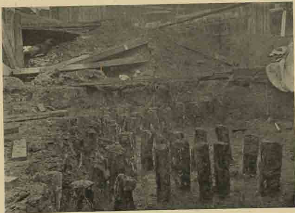
Fig. 3. Westminster Belfry : piles under raft.
