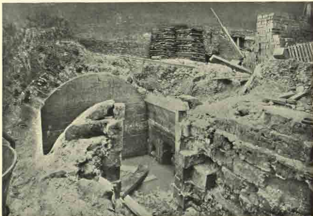
Fig. 1. Queen Square: Interior of reservoir after removal of vaulting
