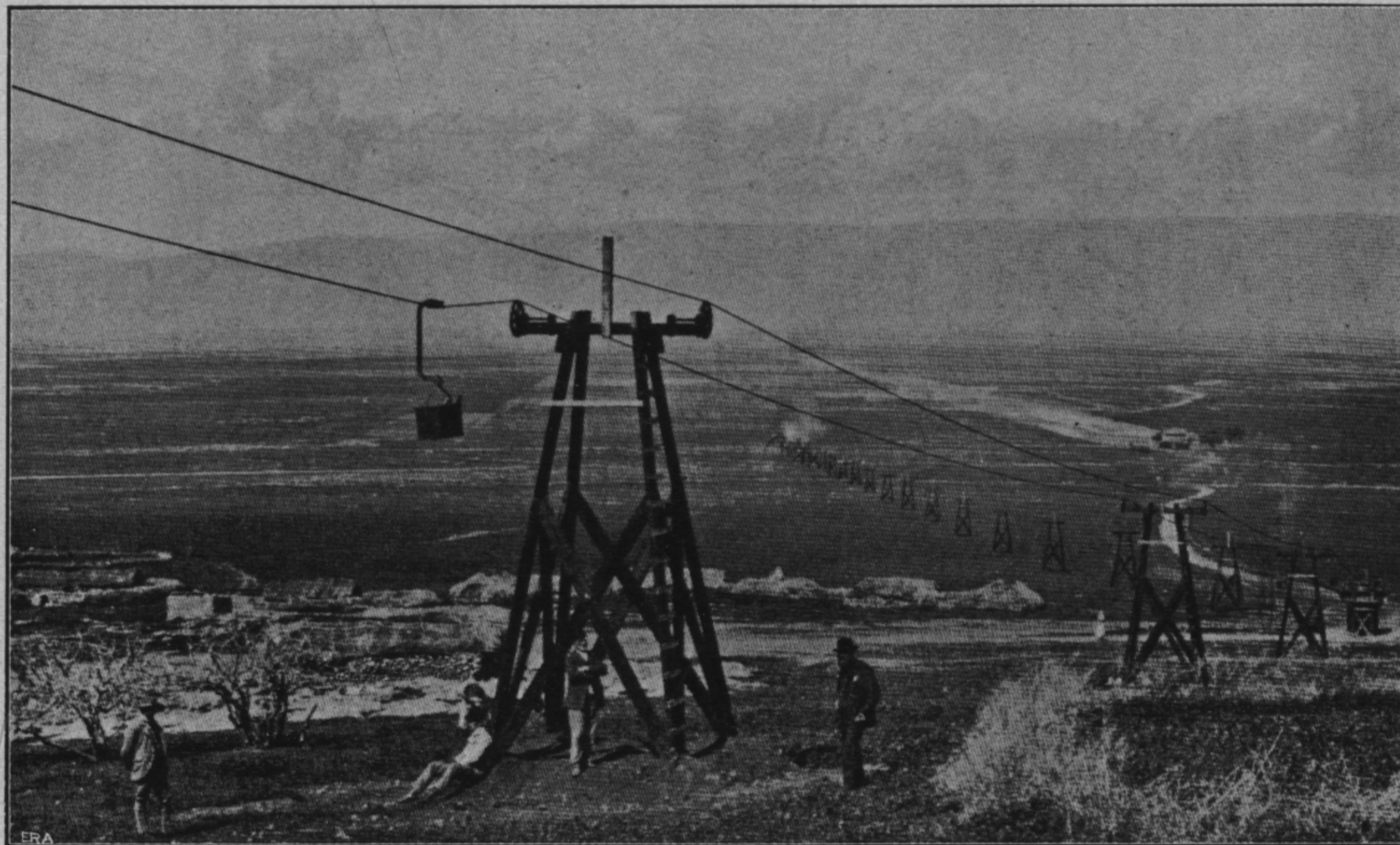
FIG. 46.—Installation of Wire-Rope Tramway in Algeria : Angle and Portion of Line.
