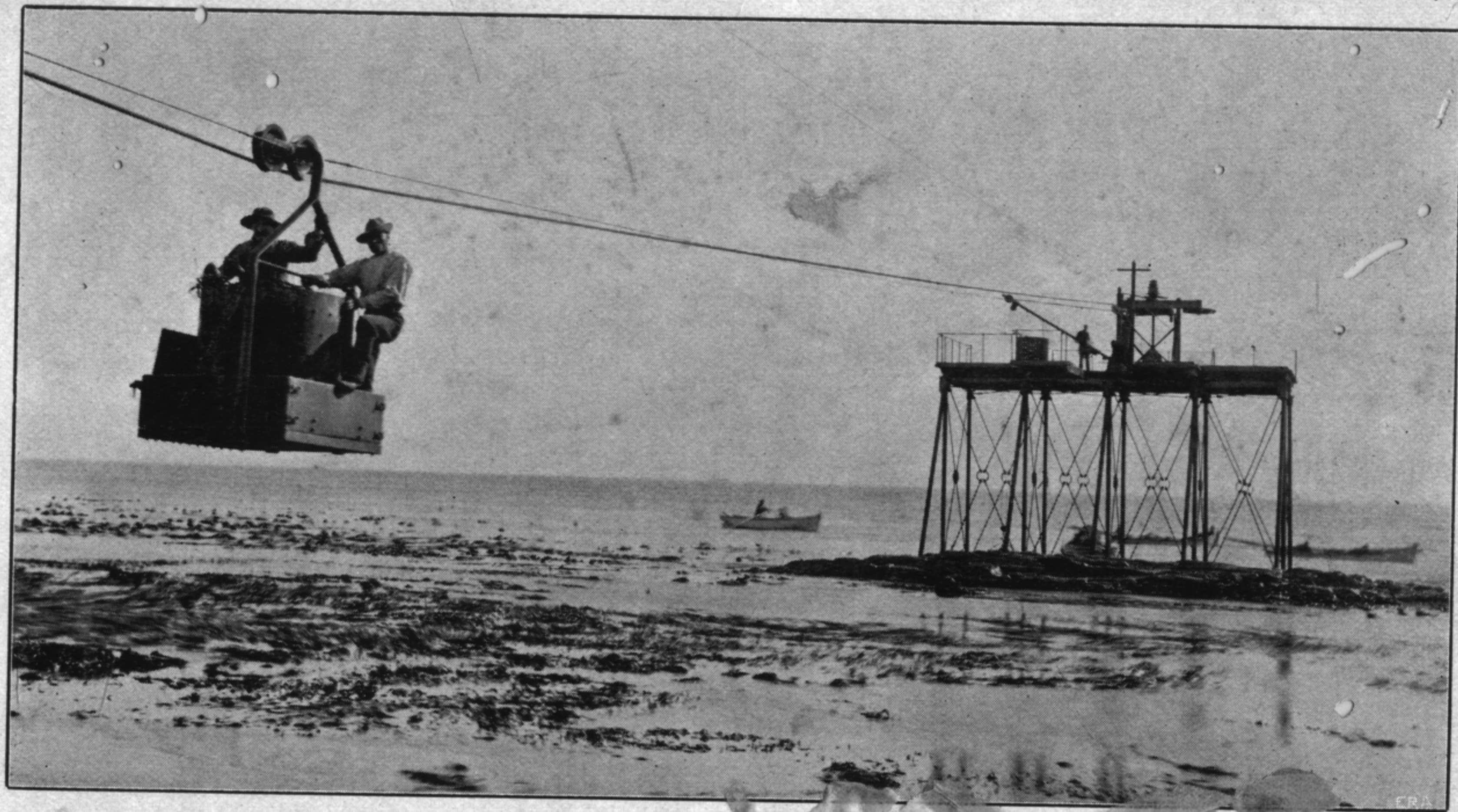
FIG. 75.—Installation of Wire-Rope Tramway as Pier in the Bay.
