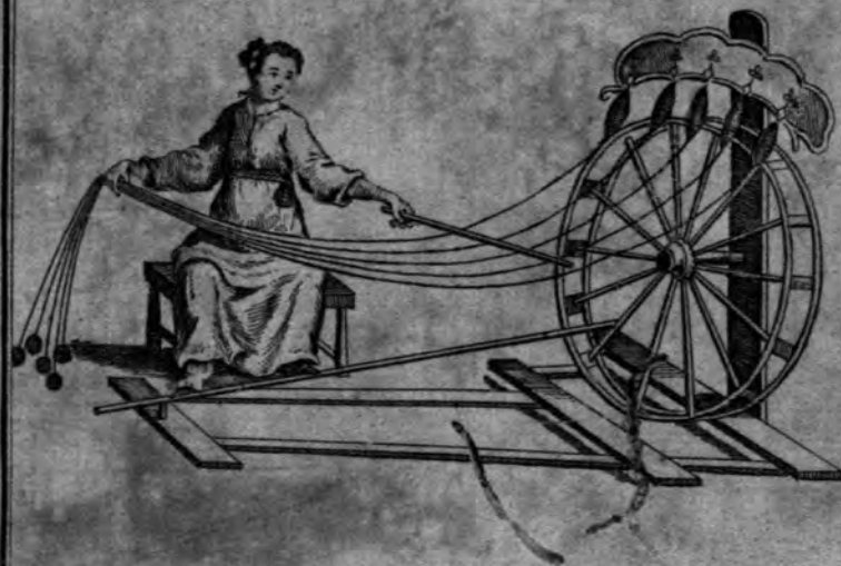
Winding from the Clews to the Bobbins.
