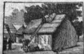
METHOD OF APPLYING THATCH.
