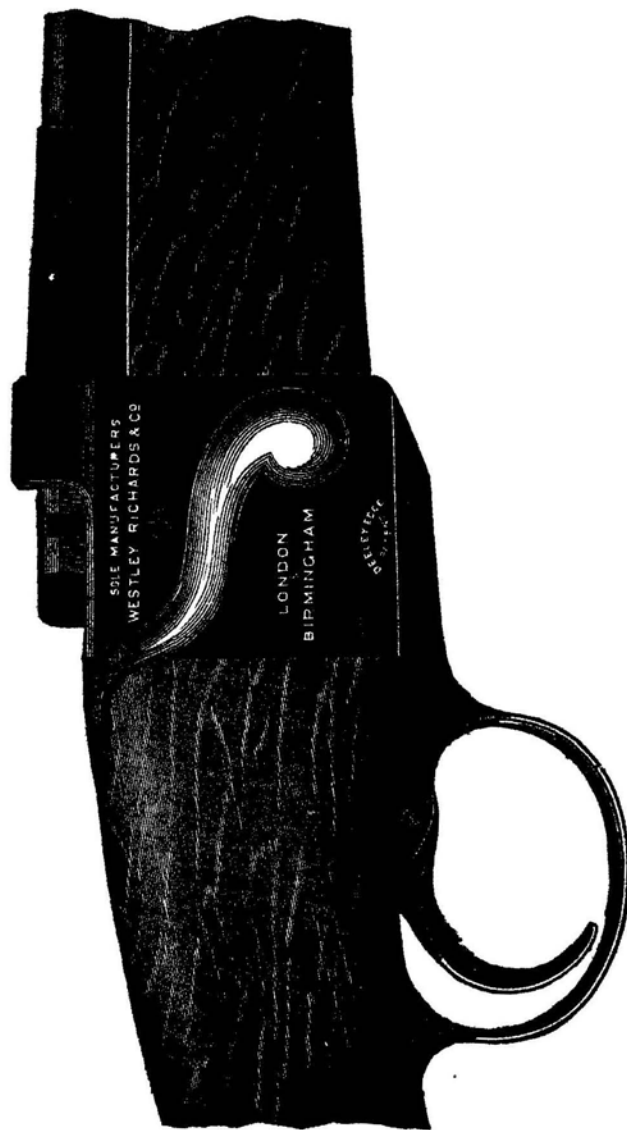
FIG. 184. EXTERNAL VIEW OF DEELEY-EDGE-METTFORD RIFLE, SHOWING BRANCH ACTION.
