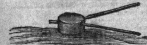
fourteen or fifteen inches thick, with one short, and two long handles, as per sketch. A man at each of the long handles manages the fall of the beetle, and a third man by the short handle assists in raising it, to strike the blow. Such an implement was, without doubt, very suitable for *filliping* so corpulent a being as Falstaff. J. JOHNSON.
