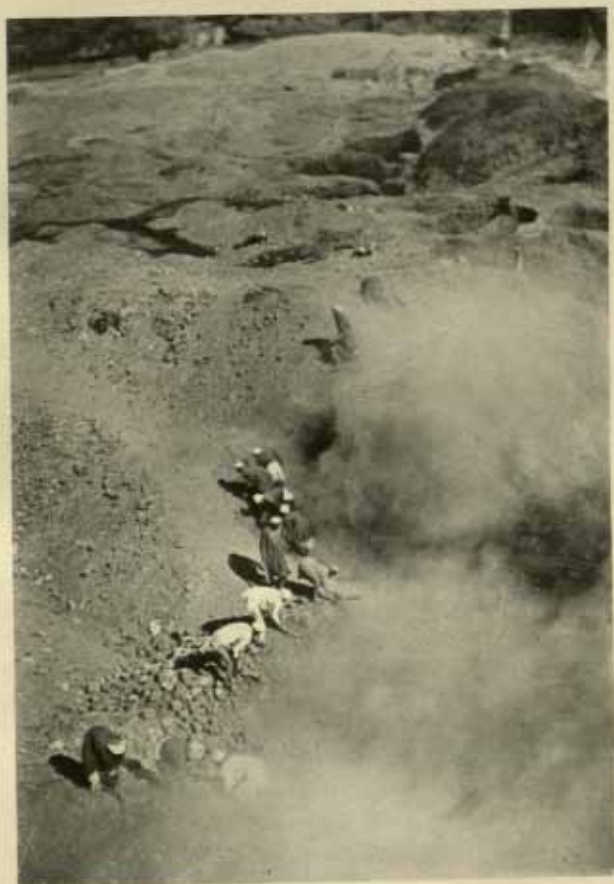
Fig. 24. CUTTING DOWN FROM THE TOP EDGE OF THE WORK.
