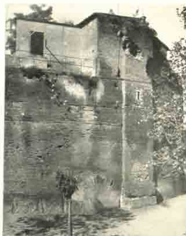
FIG. 3. N.E. ANGLE TOWER OF THE CASTRA PRAETORIA. BRICK-FACED FOUNDATION WITH RELIEVING ARCHES.
