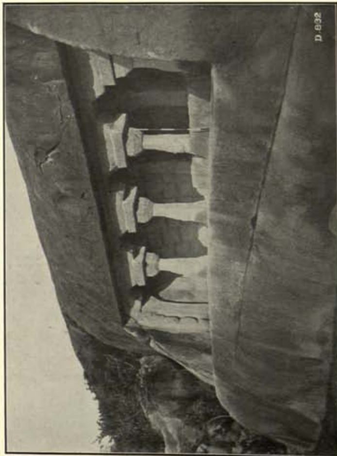
(c) METHOD OF EXCAVATION: THIRD STAGE.
