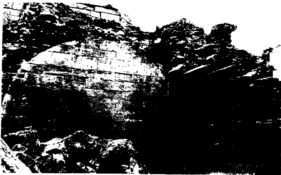
FIG. 2. Hatra, oversailing vault in main palace.
