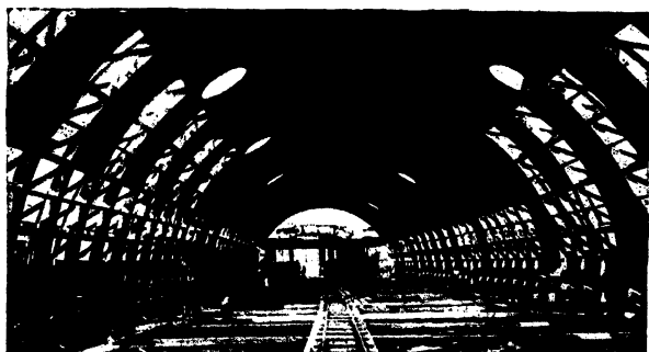
CONSTRUCTING THE METAL CAISSONS TO BE BURIED IN THE MARSHY GROUND BORDERING THE SEINE
