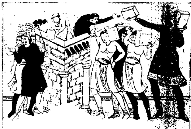
MASONS AT WORK IN THE ELEVENTH CENTURY, WHEN MANY MONASTERIES WERE BUILT. On the right they are bringing stones; and on the left they are working a windlass (note the rope).
