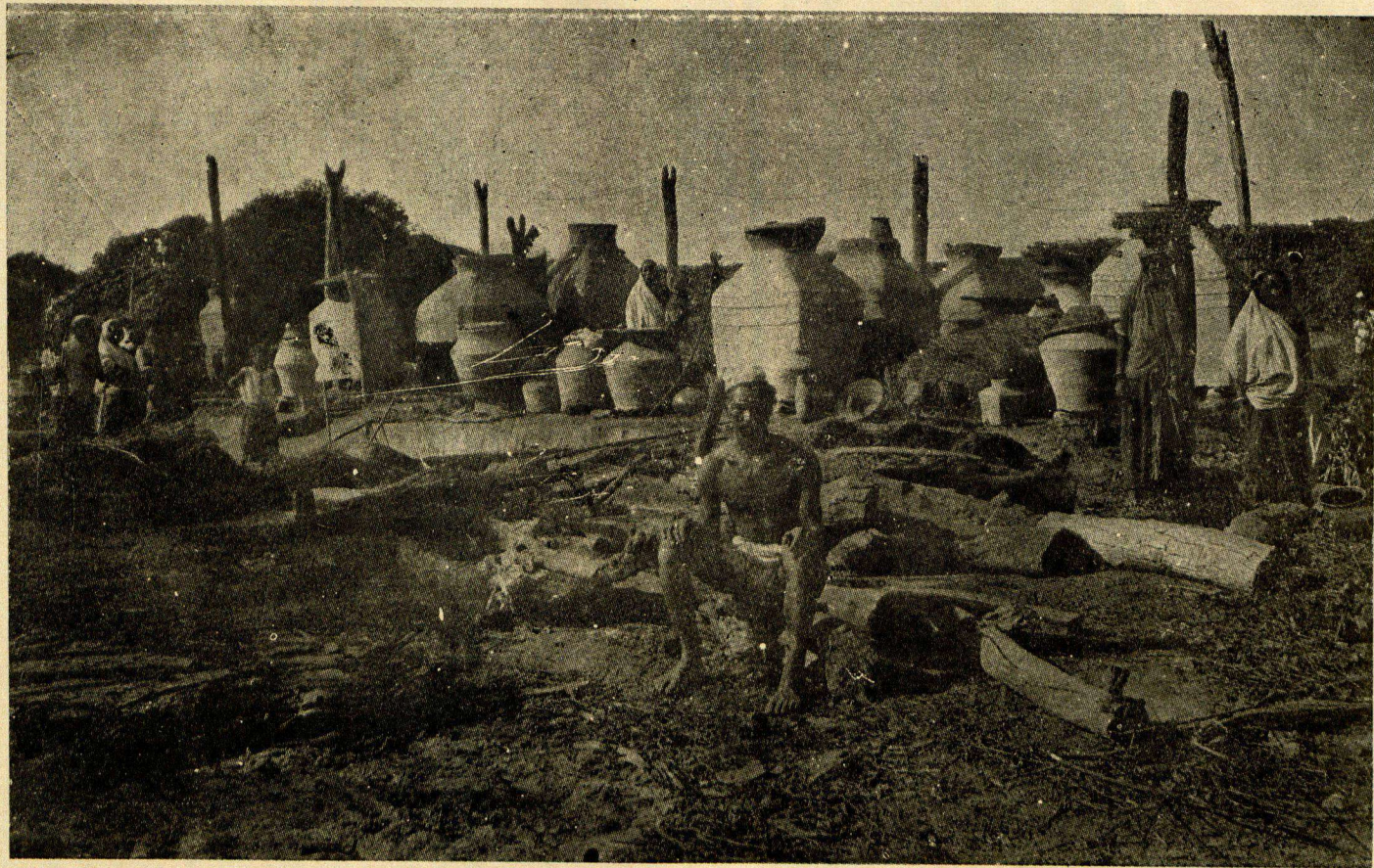
INTERIOR OF THARU HUSE, (AFTER A FIRE)
