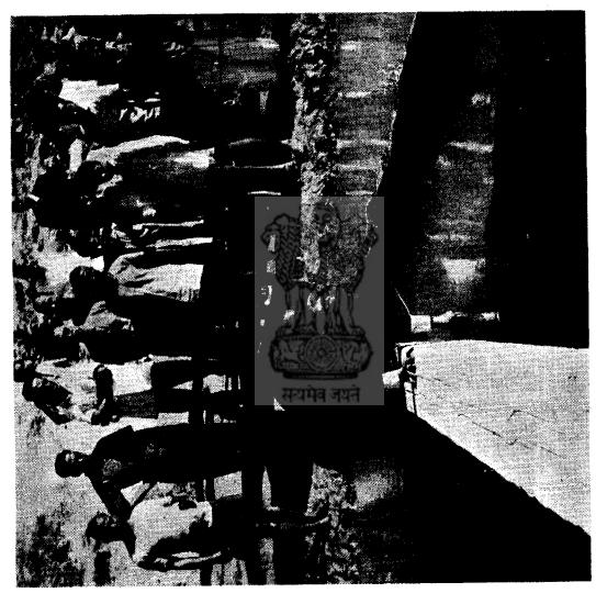
Sample of water being collected by refinery officers near the approaching plank of the Jamalpur water supply dock. The thick oil refuse can be seen in the water in the foreground of the picture. (Ex. 1—plate 1) 4.3.1968.
