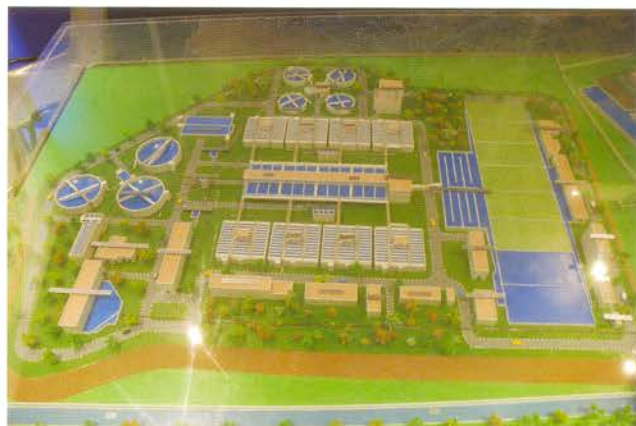
Fig. 6. Model of the Sonia Vihar water treatment plant that processes and supplies 140 million gallons of potable water per day.
