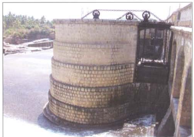
Fig. 8. Well with float and counterweight arrangement
