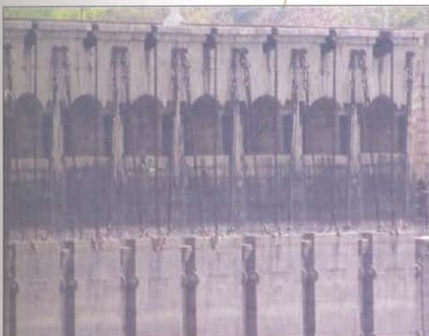
Fig. 6. Chain & Pulley arrangement for gate opening
